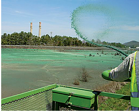
Dyed green to facilitate application and inspection
